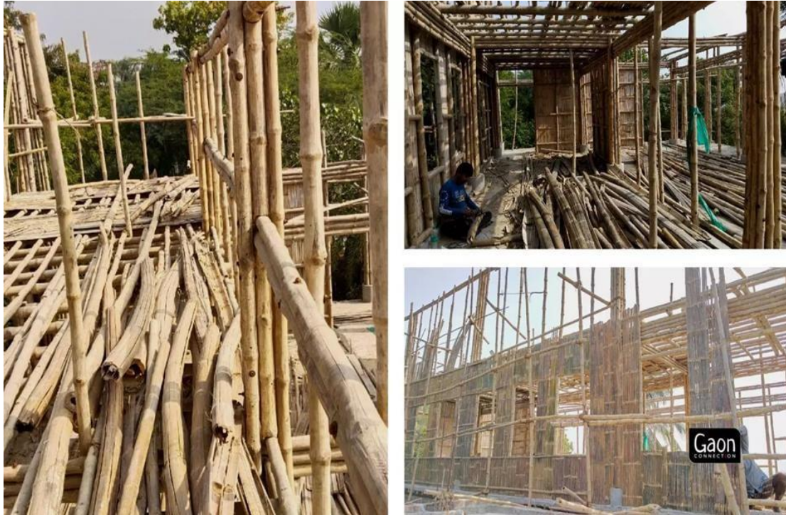
Figure 14: Construction of Stilt houses with bamboo structure on top in Sundarbans.
