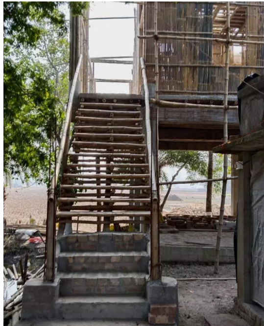
Figure 15: Bamboo combined with concrete
