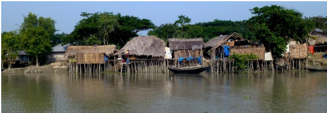
Figure 13: Stilt Houses of Sundarbans, West Bengal
